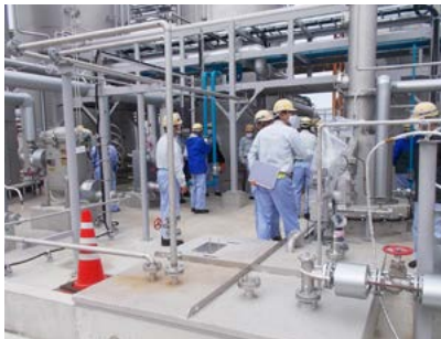
Safety audit prior to trial operation of wastewater infrastructure (Nihongi Plant, September 11, 2020)
