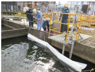
Environmental abnormality response drill (Takaoka Plant, October 7, 2020)
