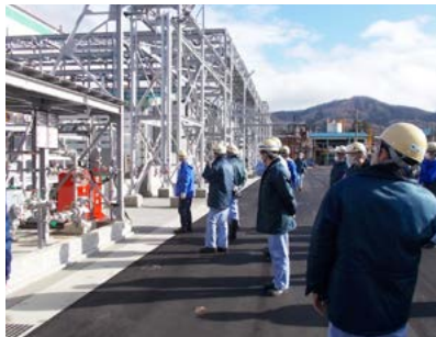
Safety audit prior to trial operation of E line of HPC production (Nihongi Plant, December 4, 2020)
