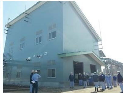
Safety audit prior to trial operation of Mg-E spherical fine particulate grade production equipment (Nihongi Plant, March 4, 2021)
