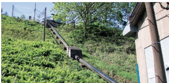
From the hydroelectric power station to the water tank
